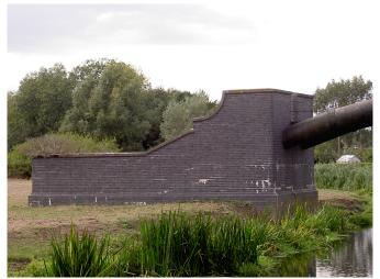
This construction is a support for the pipe where water flows over the river at the Ulting Gauging Station- one of the start points for treasure directions.
